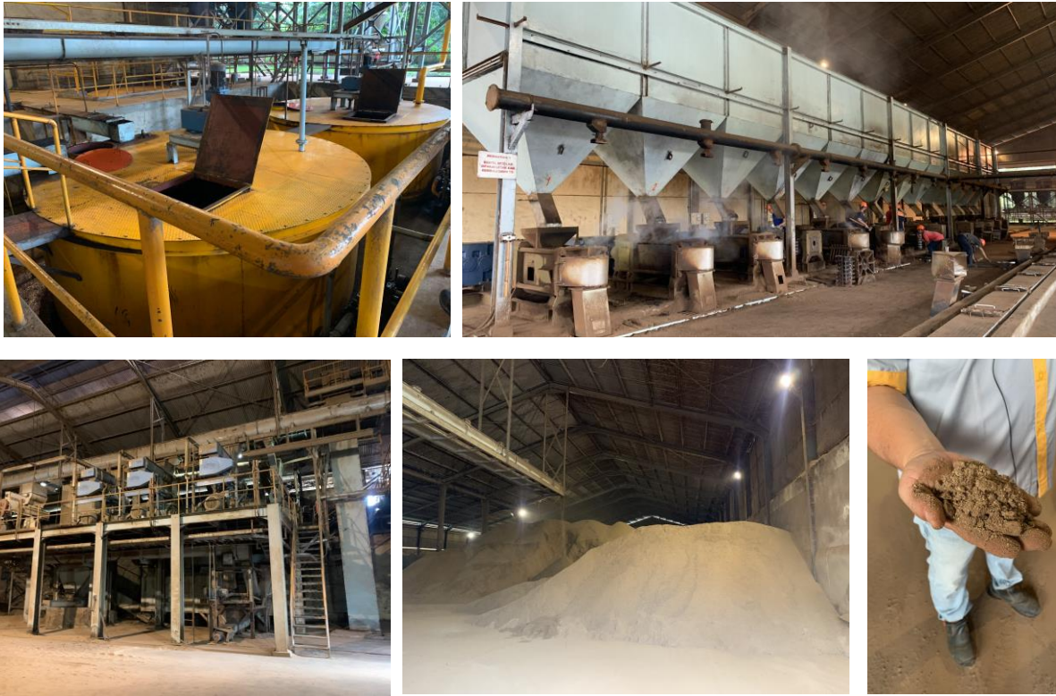
Exhibit 23. KSJA's KCP, featuring a bunker for PKM and storage for CPKO
