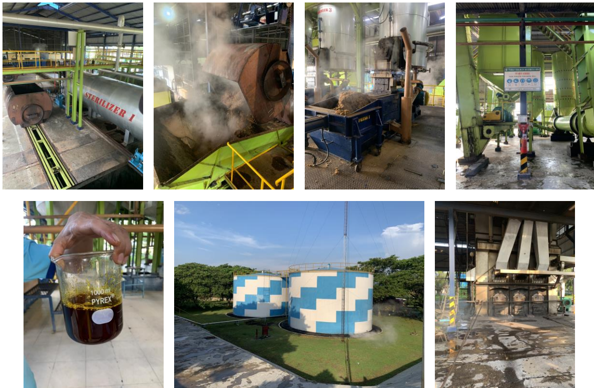
Exhibit 22. The oil mill at KSJA uses horizontal sterilizers, which can minimize losses
