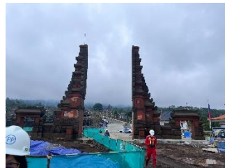
PTPP builds main road facilities in the Pura Besakih Area
