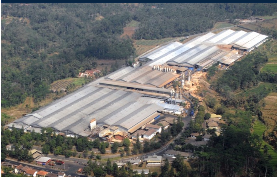
Exhibit 12. Rooftop of TKPI on which the Solar Panel would be installed
